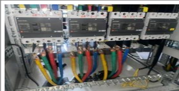
箱变低压侧电缆缺失标牌
